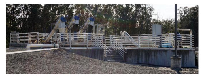
The WRF is designed to treat a buildout flow rate of 2.5 MGD at average dry weather flow conditions and 5.0 MGD at peak wet weather flow conditions. The WRF process train includes an emergency overflow basin, headworks, anoxic basins, aeration tanks with membranes, metering, and disinfection. In order to meet the projected buildout demands, the City will need to reuse 100 percent of its treated water during peak demand in the summer months.
